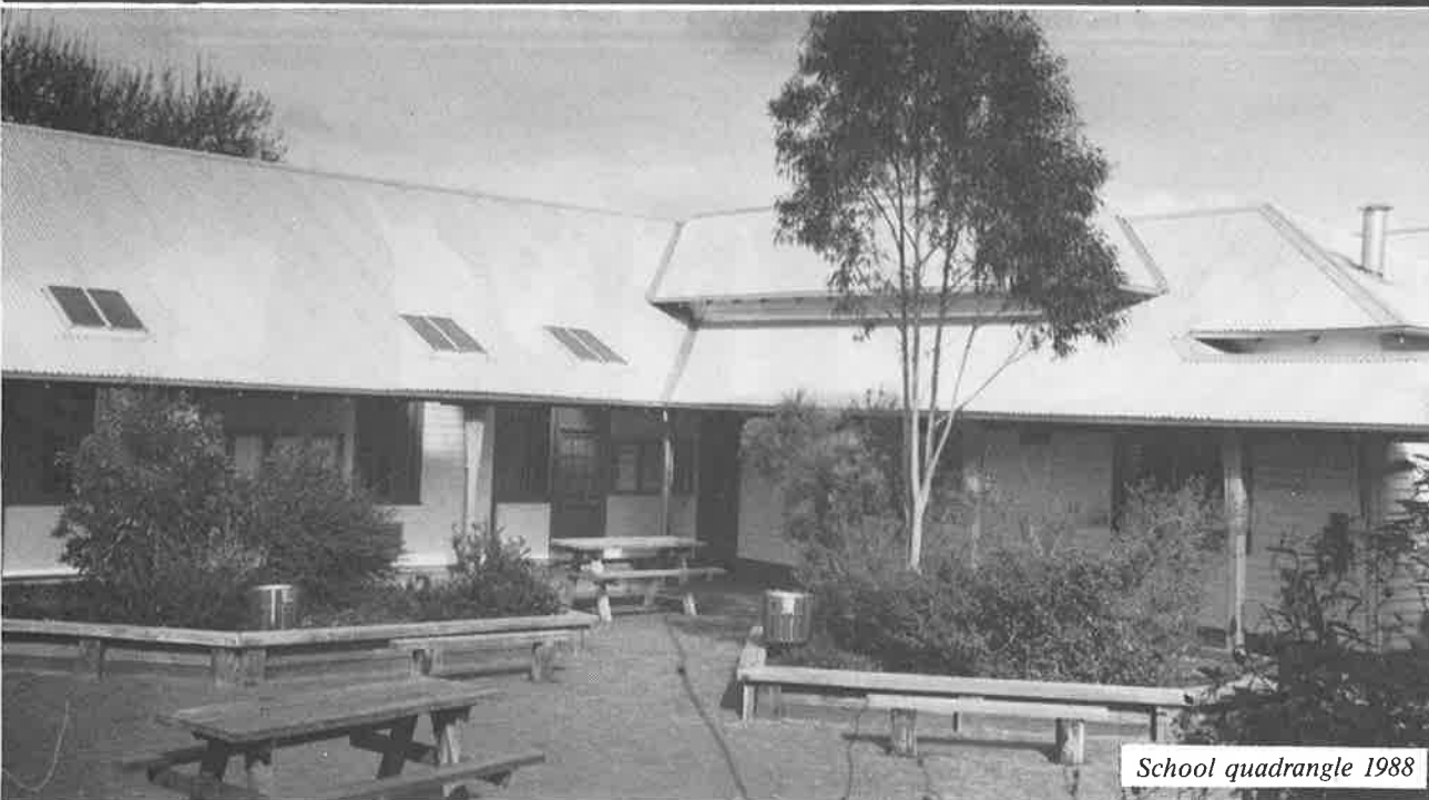
Quadrangle looking West before the upgrade
