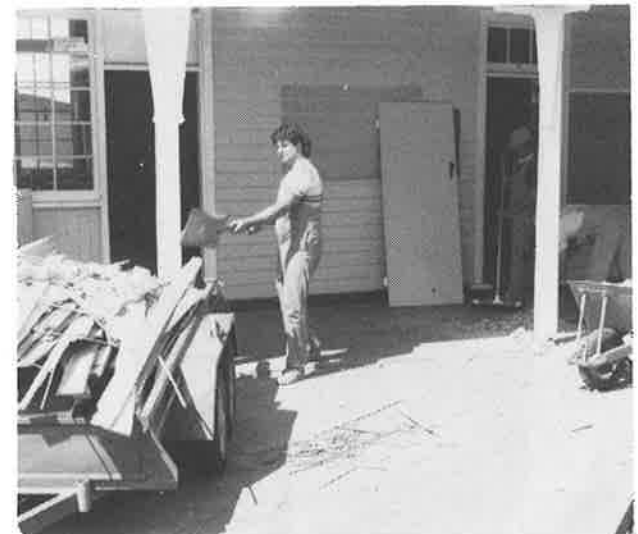
Renovations for the new staff centre 1984
